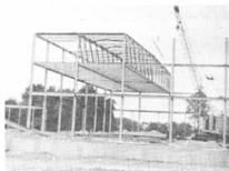
GOING UP! (Steel for Dickinson High)
